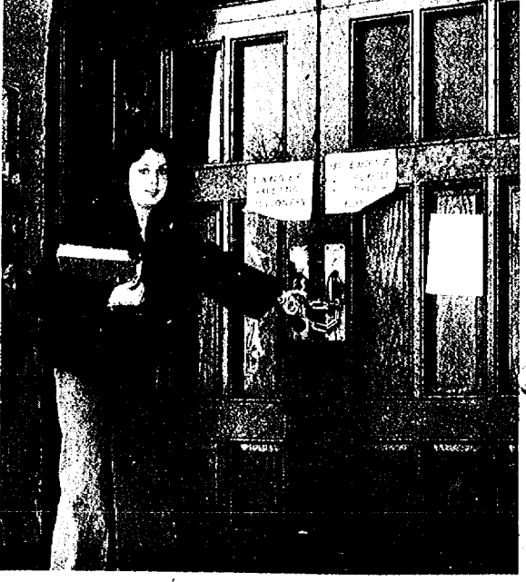
Photo by W. Kwang Locked doors because of falling masonry prevent Stephanie Mills from entering Shepard Hall on St. Nicholas Terrace.
