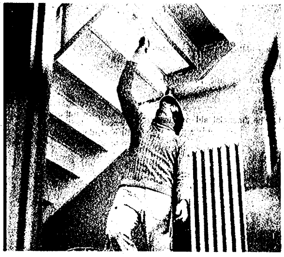
Photo by W. Kwang Painter adds final touches to Downer stairwell.
