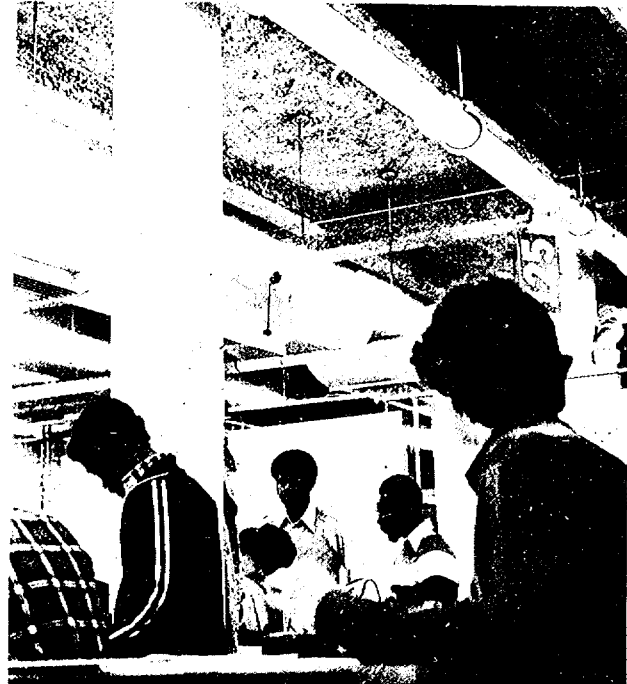
Photo by David S. Eng Students go through daily class schedules in Curry while peeling asbestos hangs over their heads.
