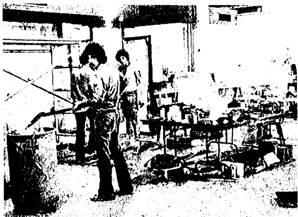
GAD/Gregory Durniak Work continues on the new Coffee house.
