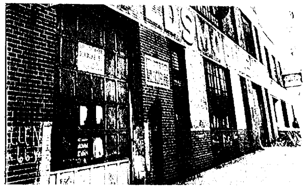
The garage, at 133rd Street between Broadway and Amsterdam Avenue, that the College plans to rent for faculty parking. Photos by Gregory Durniak
