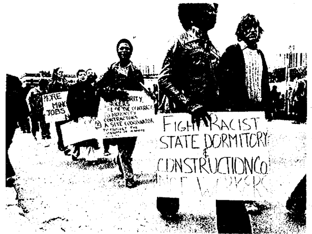
Student supporters picketing the construction site. Photos by Gregory Durniak
