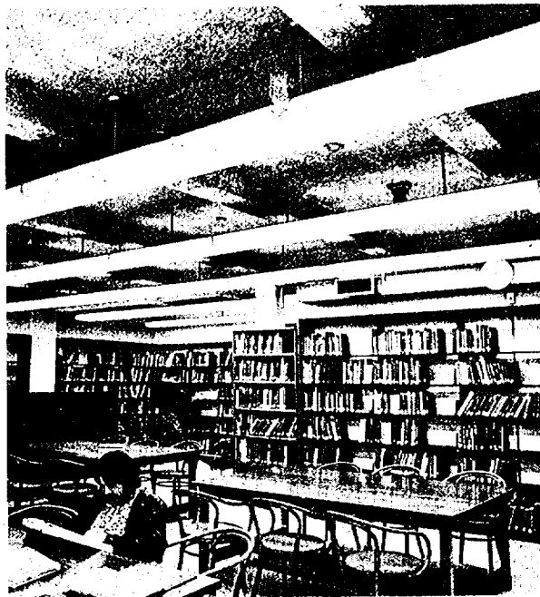
Photo by Edmond Prins A student in the Architecture Library of Curry Garage pursues his studies, apparently unaware of the potential health hazard posed by the asbestos ceiling above.
