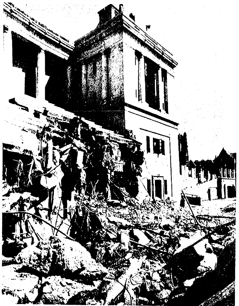
Lewisohn Stadium's north tower on Monday after start of demolition.
