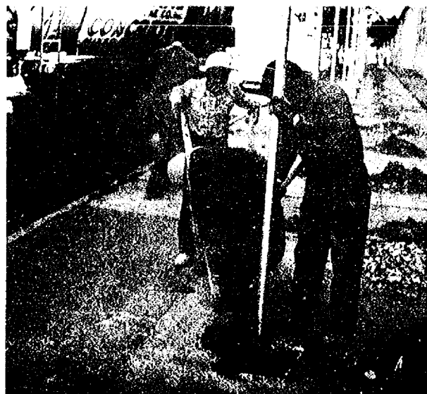
Workers secure steel posts that will support chain link fence around Lewisohn Stadium. Demolition of the Stadium is slated to begin within the next few weeks.
