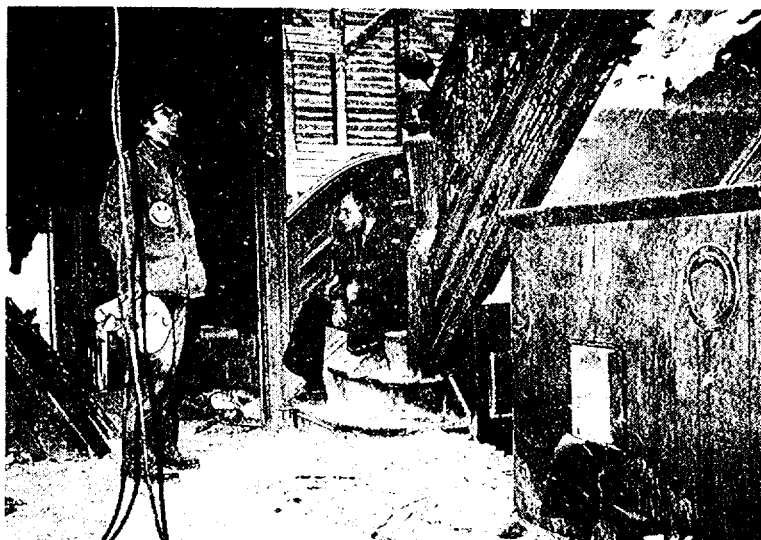
Two members of the College's Delta Alpha fraternity look over part of the $12,000 worth of damage caused by a fire that swept through the fraternity house on 143 Street during the Christmas recess.
