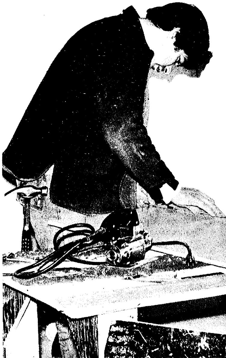
Worker saws plywood panel for one of the building's many laboratories.
