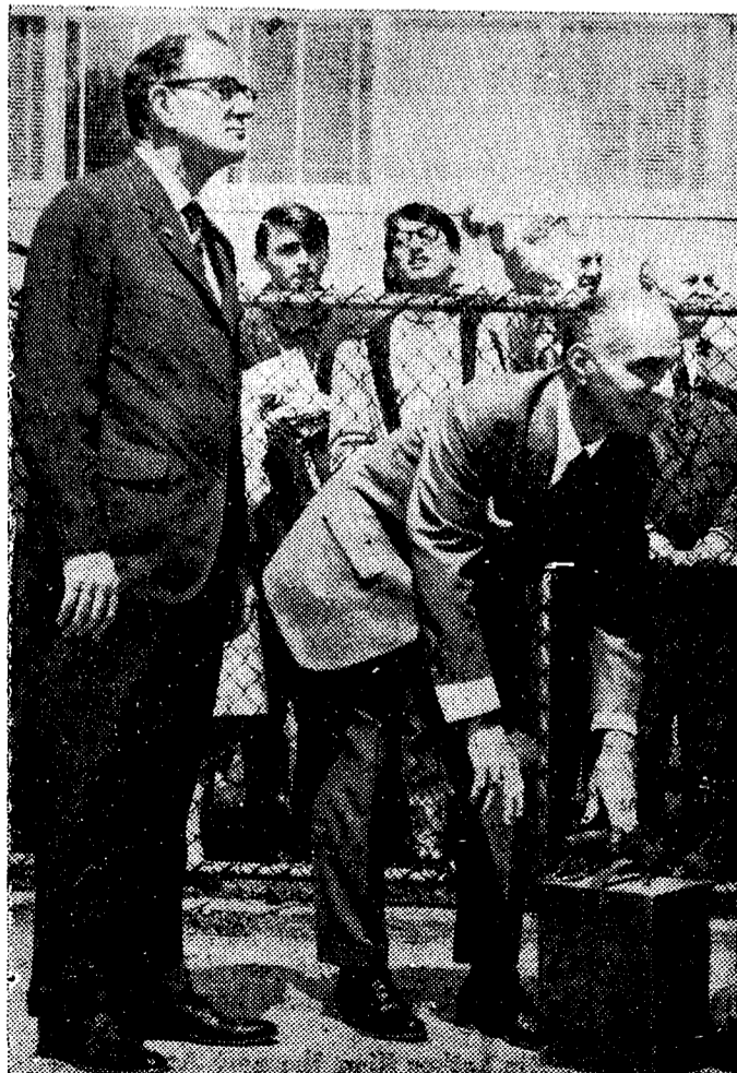
President Gallagher looks on proudly at groundbreaking for Science-Phys Ed building.
