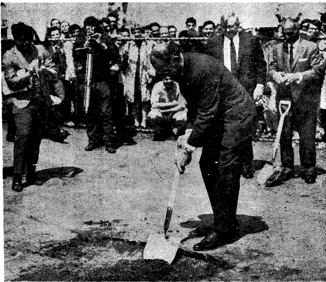
ANSWERING THE CALL OR DIG WE MUST: President Gallagher digs up first batch of dirt from Jasper Oval. New Phys. Ed complex will be initial shot in the battle of the facilities.
