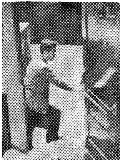
OPEN FIRE DOOR makes it easier for fire to spread.
