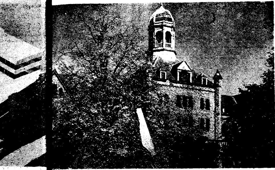
as visualized the Student Union building, currently being renovated in the plans for the renovation for its September opening. Construction is scheduled completion in May.
