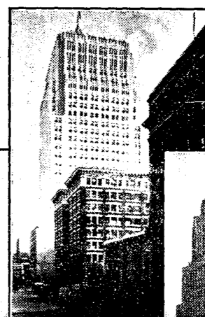
Pacific Telephone & Telegraph Company, San Francisco, Cal. J. R. Miller, T. L. Pfeuger & A. A. Cantin, Associate Architects
