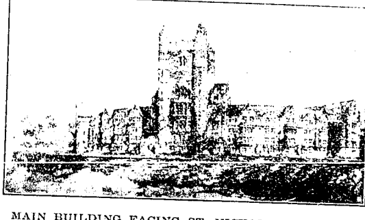
MAIN BUILDING FACING ST. NICHOLAS TERRACE
