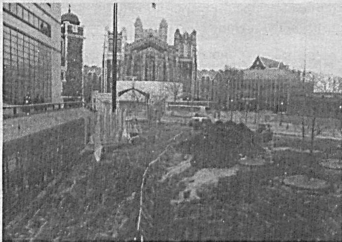
Lewishon Plaza under renovation
