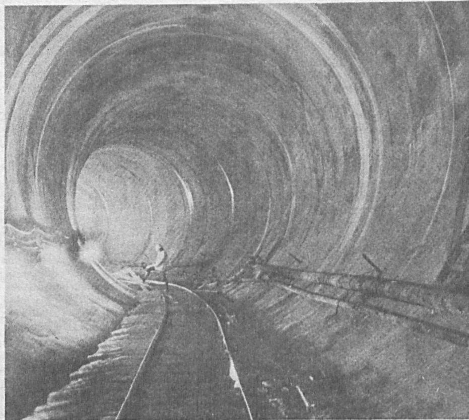
massive water tunnel 650 feet underground
